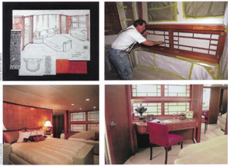
Bottom's materials and design study for the master stateroom, and the finished product. A key element in this remodeling space is the shoji screen, shown during installation, and completed. Shoji screens, one of several Oriental touches to the remodel (Alexis' owner does business in Asia), helped Bolton "square off" oval spaces back aft—without removing walls.
